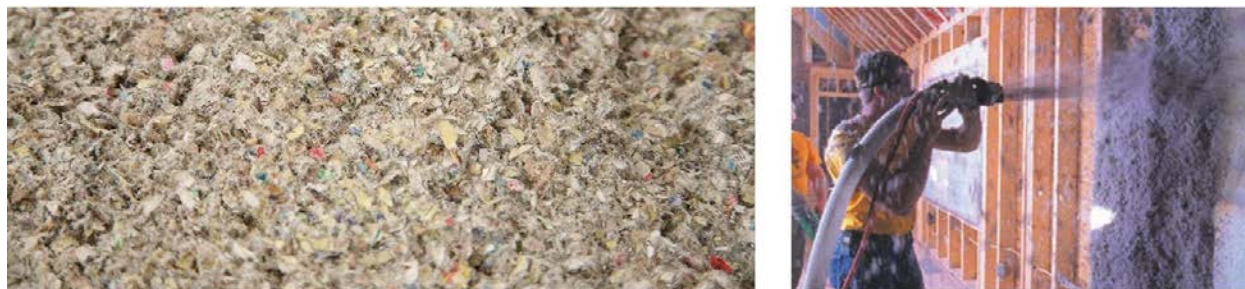
Figure 7. Cellulose spray material in closeup, and being applied.
